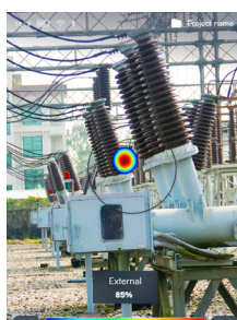
Partial discharge inspection
